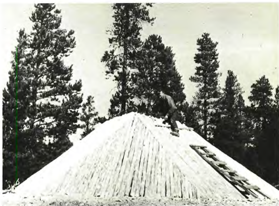
Restoration of a Chilcotin semi-subterranean house structure in Anahim Lake, British Columbia plateau. The restoration is based upon archaeological and historical evidence. In the illustration the framework has been completed and sod will be used to cover the entire outside of the house. These dwellings were entered through the roof. ( Archaeological Survey of Canada )
